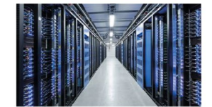
Starting at Data Center
